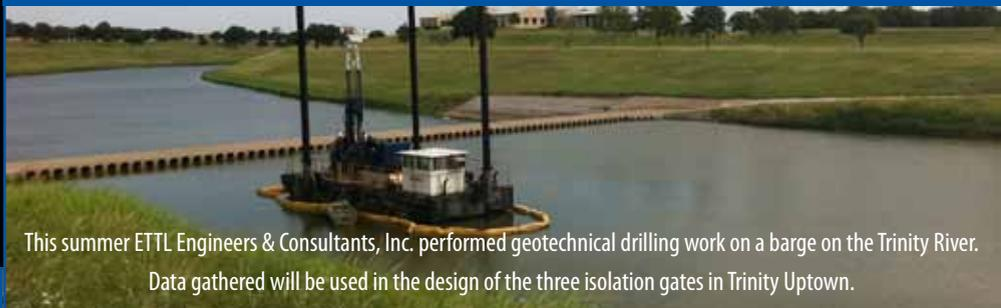
This summer E TTL Engineers & Consultants, Inc. performed geotechnical drilling work on a barge on the Trinity River. Data gathered will be used in the design of the three isolation gates in Trinity Uptown.
