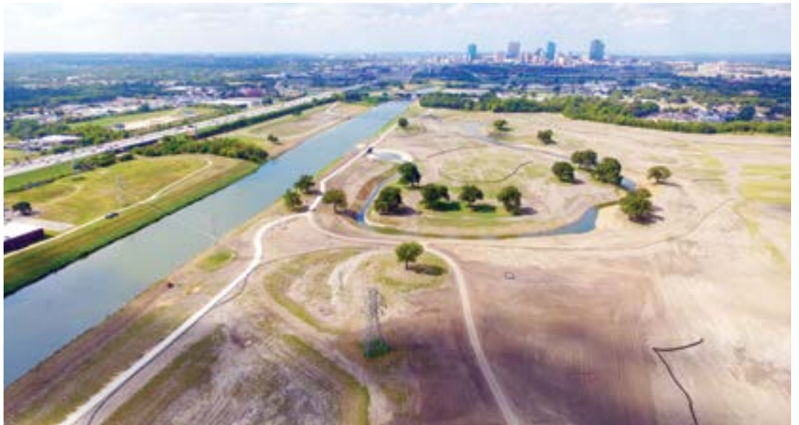
Excavation work completed to date at Gateway Park
