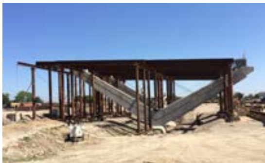
Bent 5 falsework being installed at White Settlement
