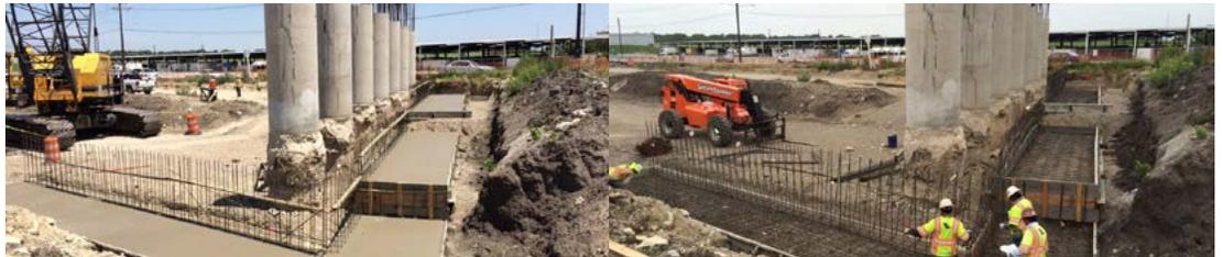
Henderson Street Bridge - Steel Being Placed for Cast-In-Place Retaining Walls
