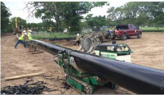
Water and sanitary sewer work in Gateway Park West – crews fusing the high-density polyethylene pipe.
