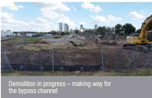
Demolition in progress – making way for the bypass channel
